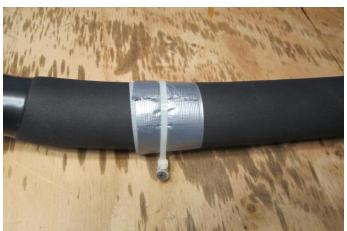
The duct line needs to be supported or it can crack the manifold and cause leaks. Wrap a couple of layers of duct tape before installing the zip tie strap to avoid damaging insulation.
