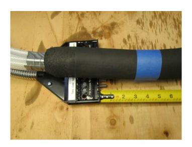
Locate duct line to Manifold and mark where to shorten insulation 5" from the manifold
