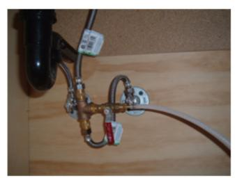
Remove the cold water flexline from the sink. Reconnect it to the tap assembly, and connect the new flexline to the sink.
